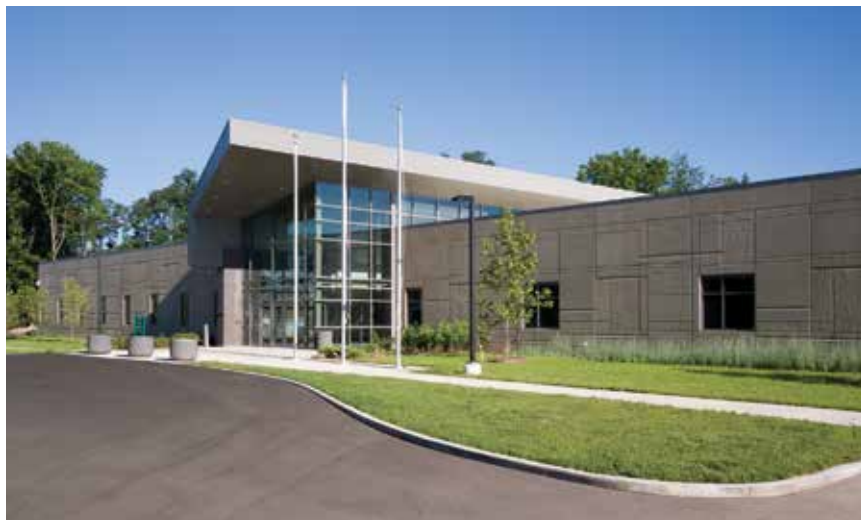
The Ivy Tech Community College campus in Elkhart, Ind., was designed by the design-build team of Ratio Architects and the Hagerman Group. The $16.8-million academic building and community center, which is clad in architectural precast concrete panels, achieved Silver LEED certification. Photos courtesy of MV2 Photography
