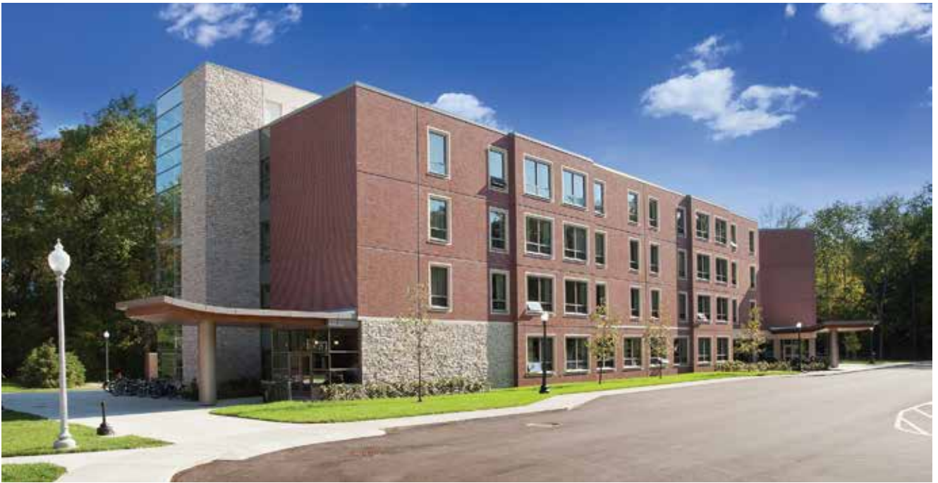
The new Residence Hall at Rose-Hulman Institute of Technology in Terre Haute, Ind., completed in 2012, features architectural precast concrete insulated panels embedded with thin brick. The 70,000-square-foot, 240-bed facility was the first facility on campus to achieve Silver LEED certification.
