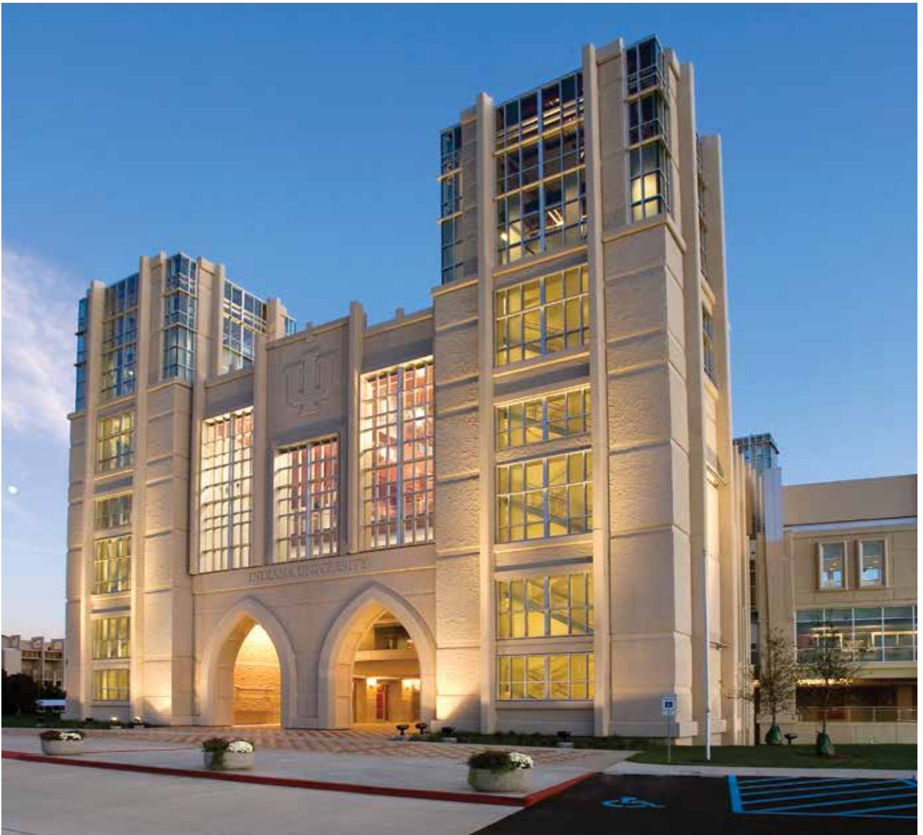
Ratio Architects created a north end-zone addition to the venerable Memorial Stadium on the Bloomington campus of Indiana University using precast concrete panels to create a Gothic style that blended with the limestone-clad buildings throughout the campus. Grandstand bleacher seating also was replaced with permanent precast concrete seating.
